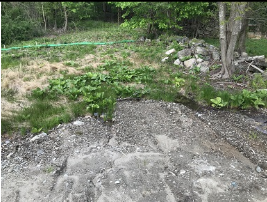
Location of the lower end of the infiltration basin. Note water and skunk cabbage indicating poor soils and high water table. 5-12-21
