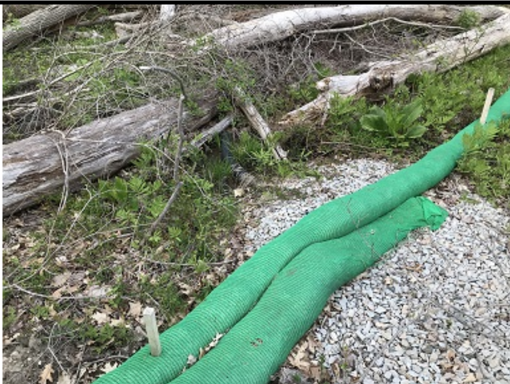
End of stone trench and 4 inch pipe past sediment barrier. 5-12-21
