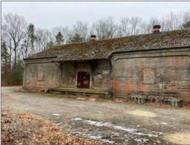
Existing Building on site (to be removed)
