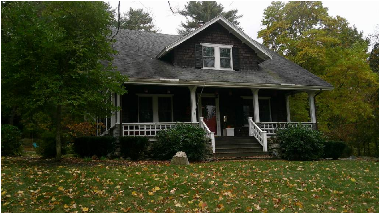
PHOTO 1: SOUTHERLY VIEW FROM ABOVE LEACHING FIELD
