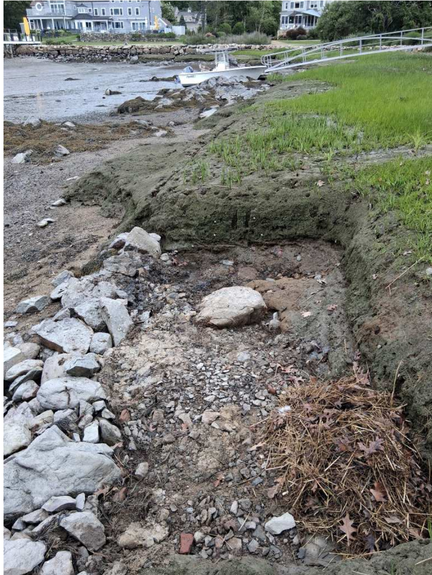
Float-damaged area with stakes, filter fabric and other debris removed.
