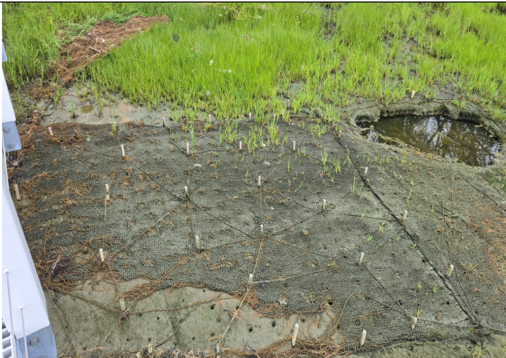
Seaward edge of southern side of salt marsh restoration area. Plantings toward seaward edge too low to thrive.
