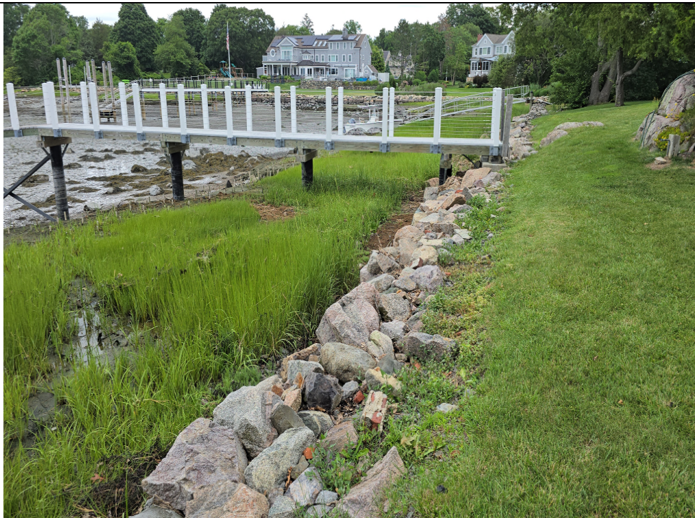
Main area of salt marsh restoration area on south side of dock. Plantings are thriving.
