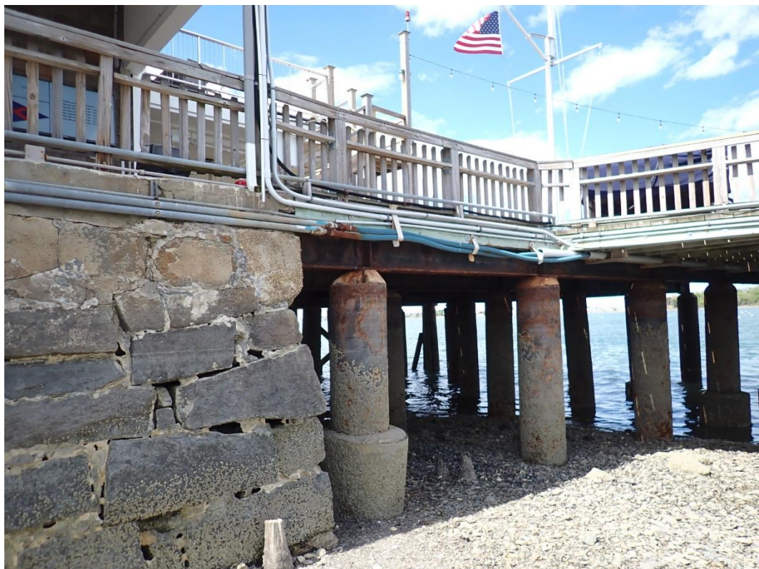
Photo 8 – East section of pier reconstructed in 2007 with concrete-encased steel H-piles.
