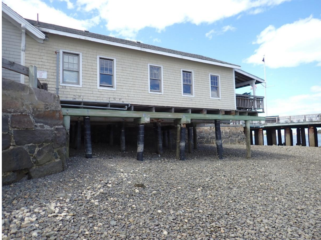
Photo 7 – One-story pile-supported pier structure with locker rooms and junior facilities.
