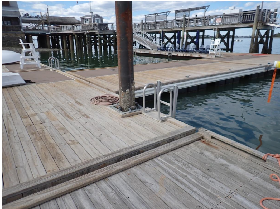
Photo 6 – Timber floating dock with steel guide pile looking northeast.
