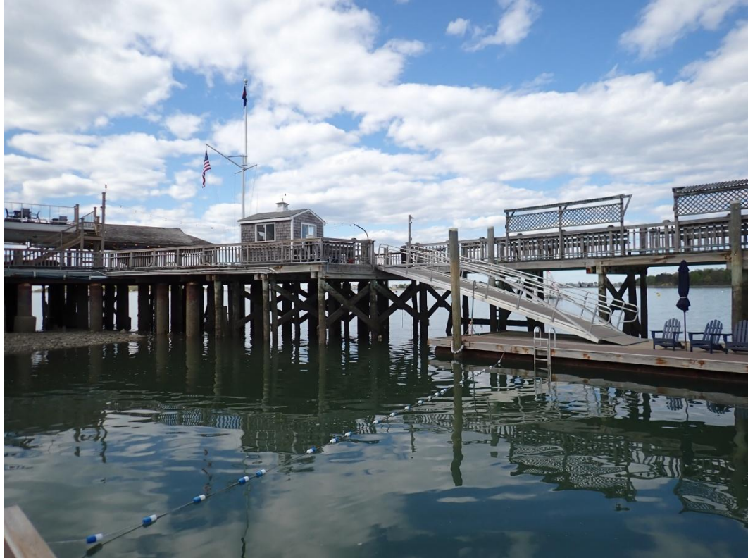
Photo 3 – East pier and finger pier looking northeast across swimming area from floating dock.
