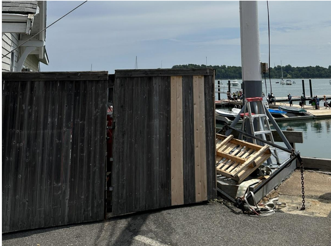
Photo 13 – Existing trash enclosure next to locker room building that will be removed.
