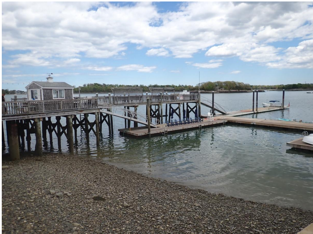
Photo 4 – East pier, finger pier, and floating docks looking southeast from deck.
