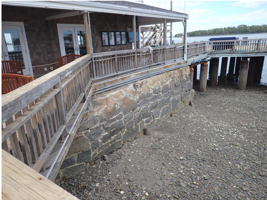
Photo 2 – South side of main clubhouse looking northeast from deck.
