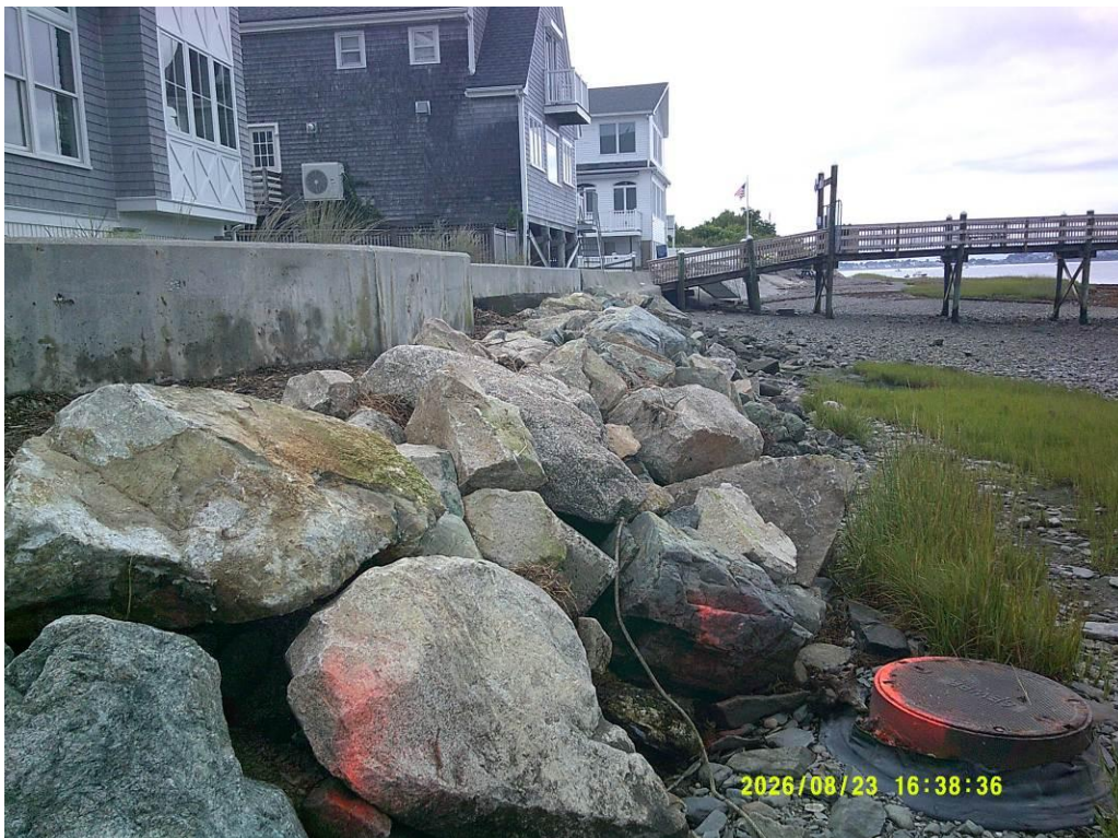
Photograph #2 – View west across the revetment restoration area.
