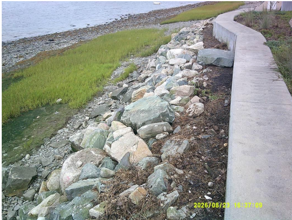
Photograph 1 – View east across the revetment restoration area.
