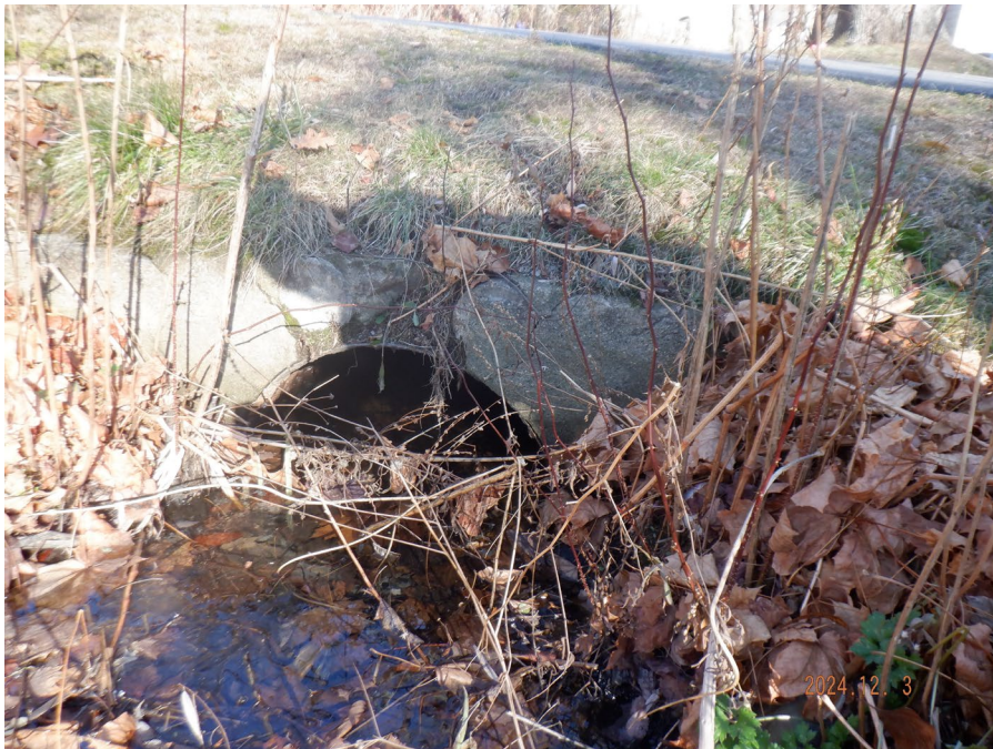
Photograph 4: View of concrete headwall, culverted intermittent stream over the southern section, facing north/northwest.
