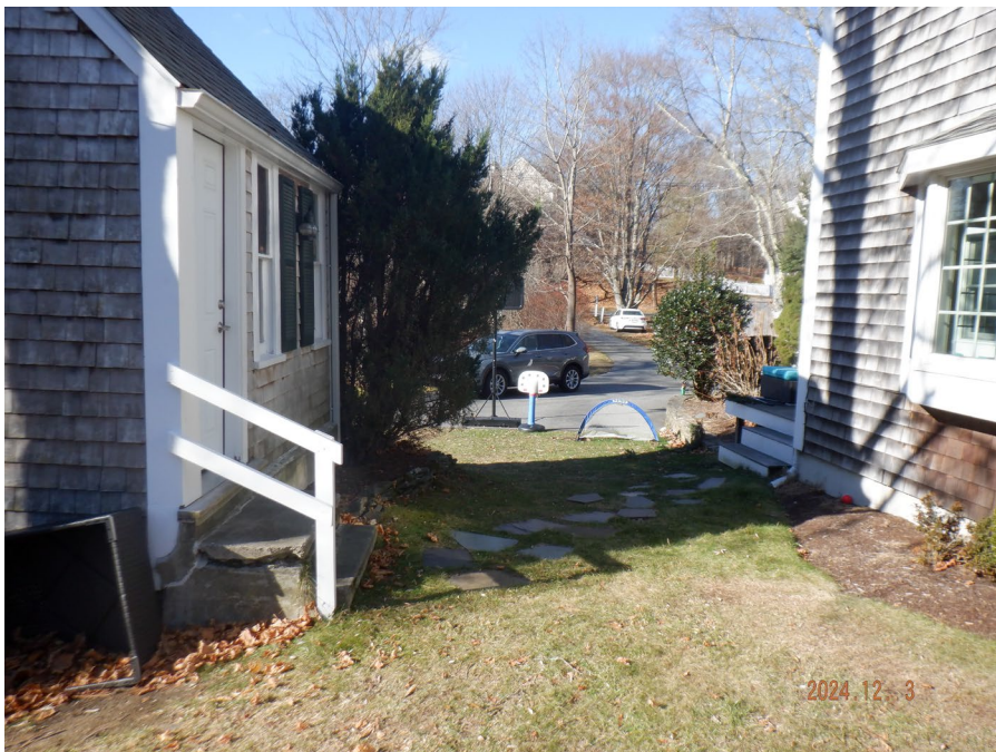
Photograph 8: Existing detached structure on a foundation (left) to be removed and proposed addition will be attached to the residence on the right.
