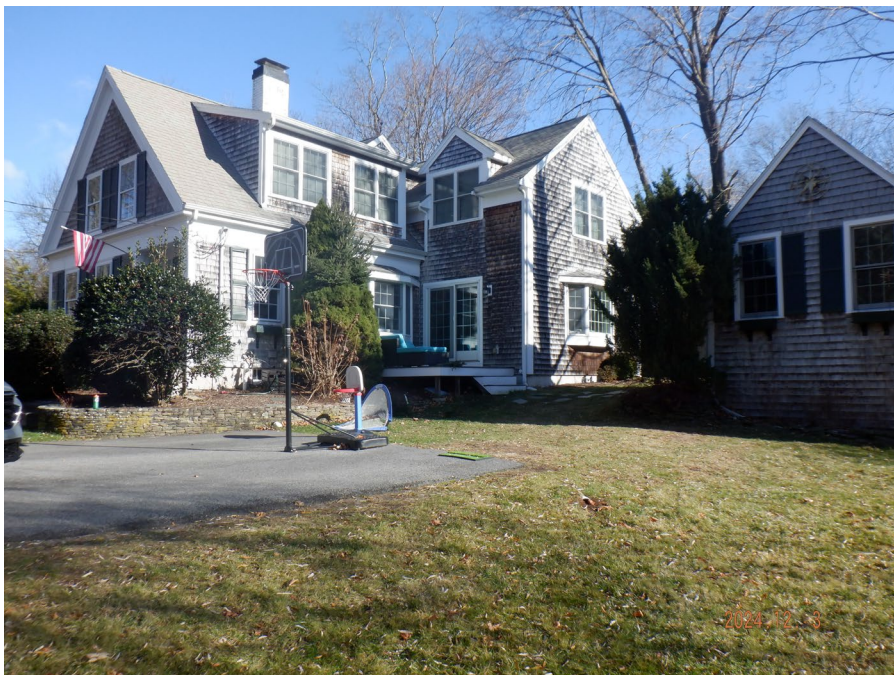
Photograph 6: View of proposed area where driveway will be extended, deck will be removed and a detached addition will be constructed.
