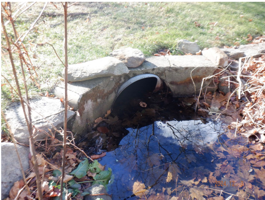
Photograph 2: Existing culvert stream pipe along northern section of Inland Bank facing south.
